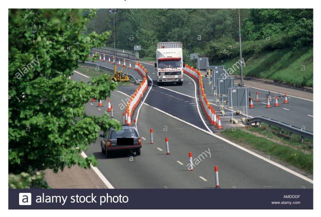
Once traffic is on the opposite side of the dual carriageway, exit lanes become a problem and invariably an extended route is required to facilitate leaving the carriageway at a junction. In the case of the A303 Westbound, should the lorry in the photograph above, be heading West and about to enter the tunnel, but wishes to exit at Longbarrow to access the Army camp at Larkhill (for example), it would have to travel as far as Wylye to exit and come back via the surrounding villages.
